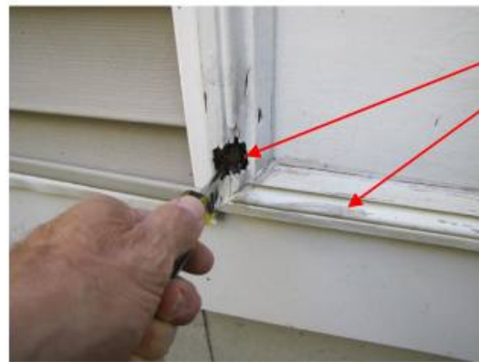
Apparent damage to metal trim and dry rot in wood trim and paint peeling
