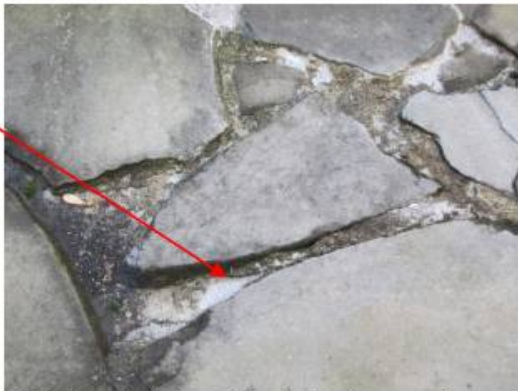
Mortar deteriorating in between stones and voids in mortar where rain water can enter
