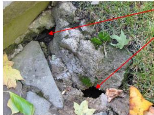
Mortar deteriorating in between stones and voids in mortar where rain water can enter
