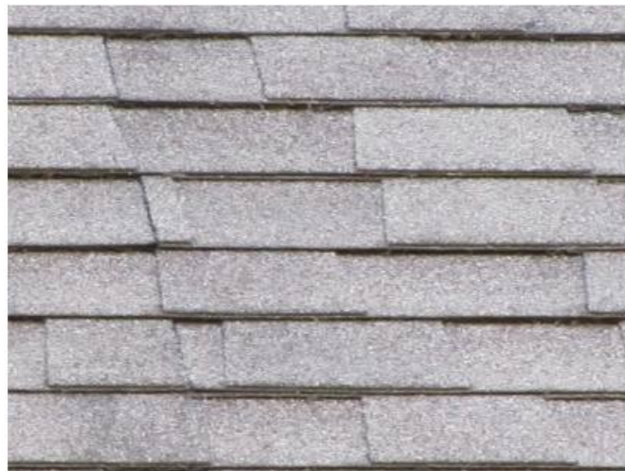
Architectural style asphalt roof
