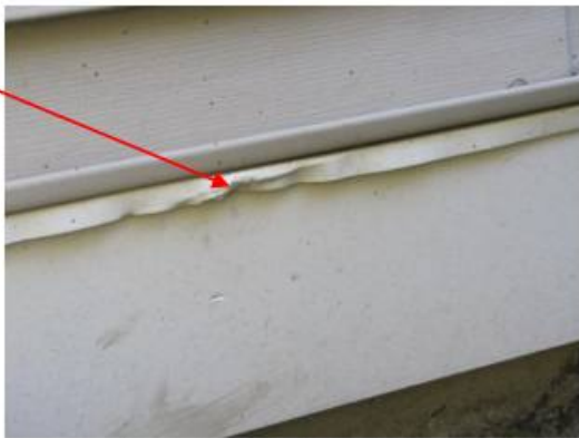
Apparent damage to metal trim and dry rot in wood trim and paint peeling
