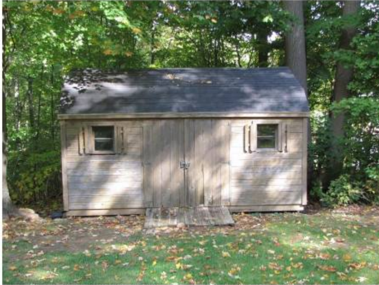
Wood shed in need of a fresh coat of stain and tree trimming
