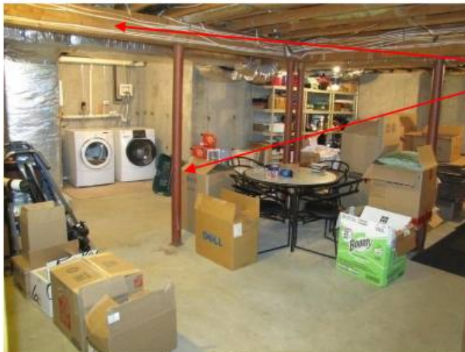
Full unfinished basement showing metal lolly columns and main carrying beam
