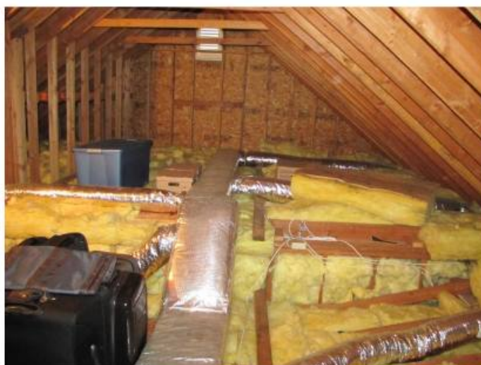
Attic showing 2X8 framing, stored items, fiberglass insulation and insulated ductwork
