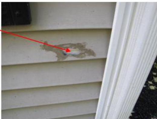
Apparent damage to siding material and staining on siding
