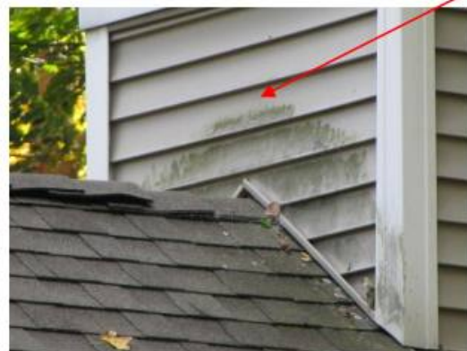
Apparent damage to siding material and staining on siding
