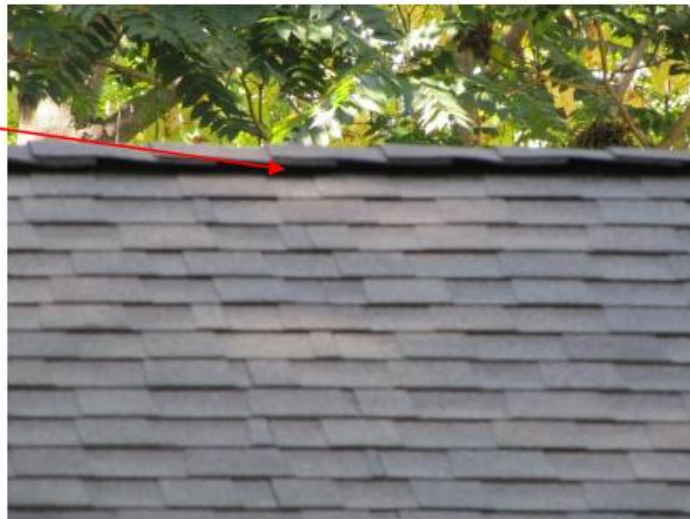
Ridge vent as seen from outside the fireside room
